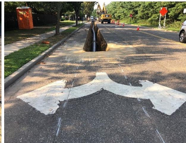
1. Segment of asphalt is cut and trench is created working around existing underground utilities
