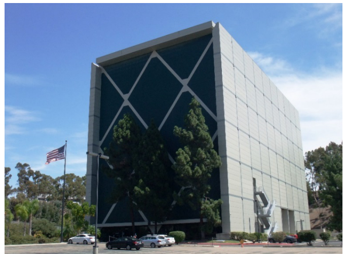
NGAS Rancho Bernardo Compact Range Facility
