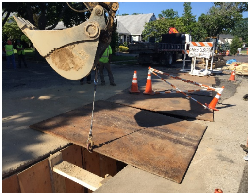
Road plates cover trenches
