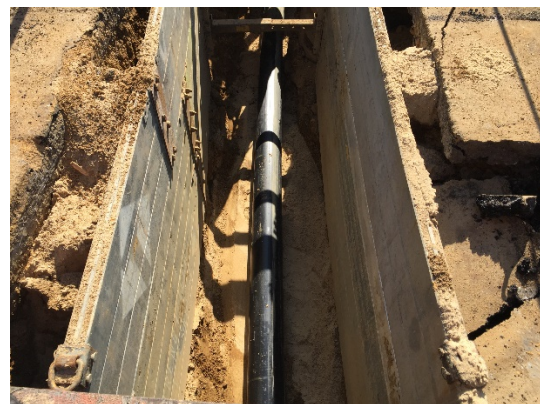
Example of pipe in trench
