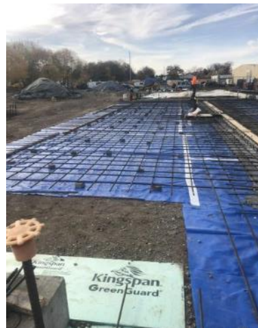
Rebar Installed for Building (Northern Floor Trench)
