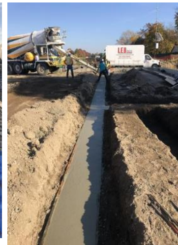
Concrete Base for Building (Southern Floor Trench)
