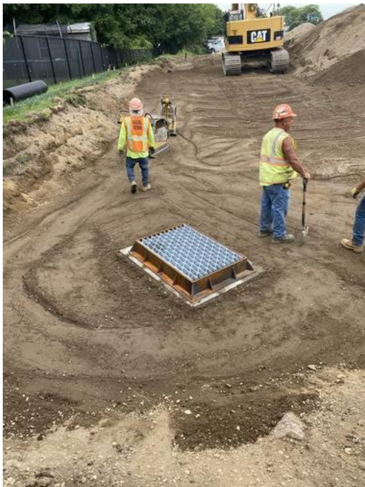
Top of Storm Sewer Catch Basin (CB-5)
