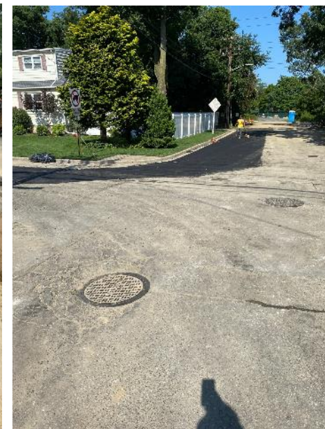
Temporary paving (Sophia to N. Herman)
