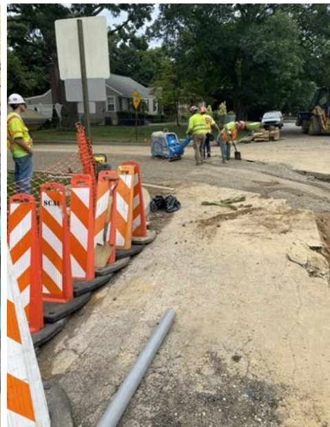
Backfill and compact road base (Sophia at N. Herman)
