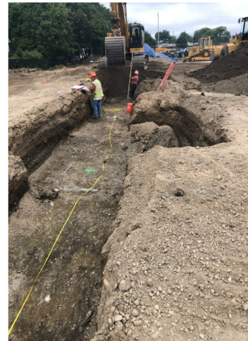
Treatment Plant Building Foundation Excavation
