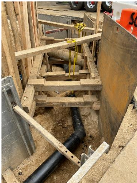
Trench and piping installation (intersection of Sophia and N. Herman)
