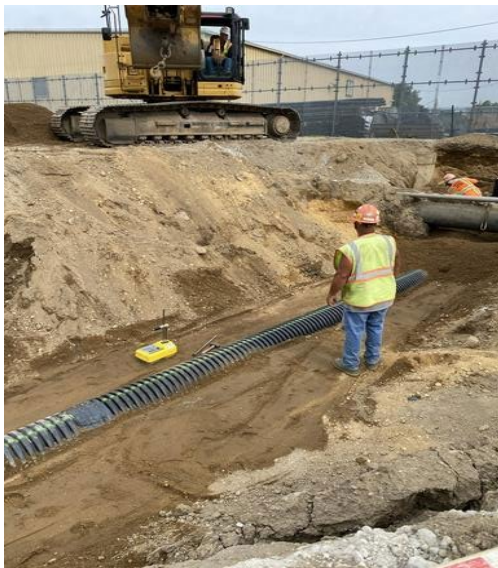
Compaction Testing of Piping Trench (between MH-1 and CB-2)
