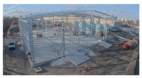
Treatment System Construction Progress: We are making very good progress on the construction of the RW-21 treatment system building. The exterior steel structure is nearly installed as are eight carbon filtration tanks. (Aerial image taken Jan 10).
