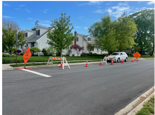
RW-20 Well location
