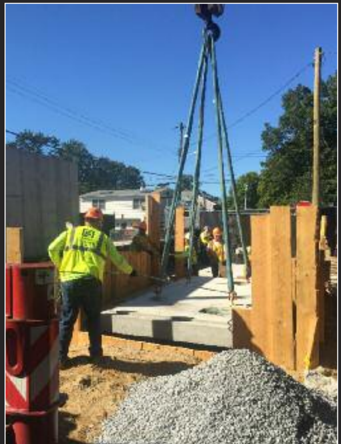
Photos courtesy of Northrop Grumman: (Left page) The men and women of Grumman Aircraft building naval aircraft during World War II. (Above, top): Grumman employees working in the clean room to assemble an Apollo lunar module in Bethpage. (Above, bottom): Northrop Grumman contractors installing a well vault for a new treatment system in 2017.
